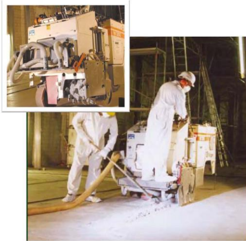
(1) Dry surface milling with dust suction
