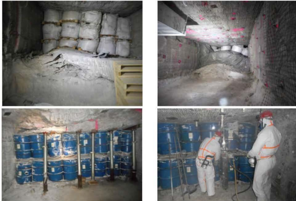
Figure 9: severely clamped packages resulting from strong rock deformations, from reference [9]
