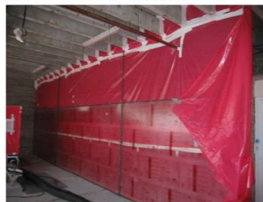
Example of physical barrier. Such material can be used to create customized locks. Source: sat KT
